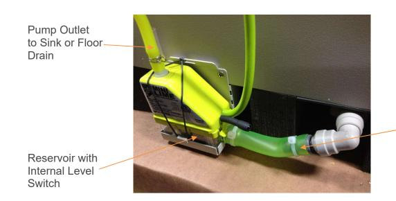
Pump Inlet from Chamber Drain
